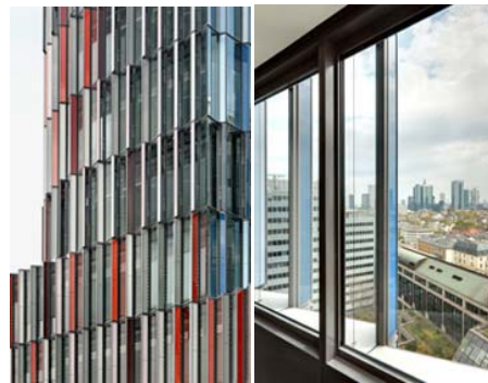
Foto 8. KFW Westerkade double-layered façade (Sumber: www.archdaily.com )
